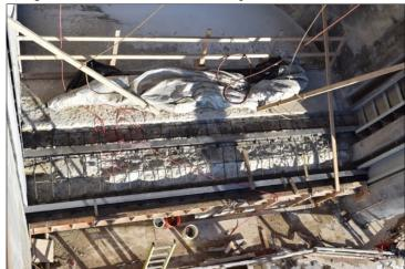
New gate guide in place along with new stop log guide in one of three rebuilt flood gate openings.
