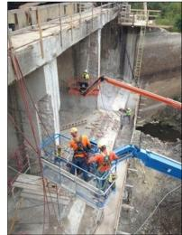
2 contractor to build the temporary cofferdam and divert the river flow through the concrete structure so the new earthen dike and overflow spillway can be completed.
