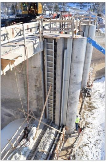
Below another picture of installed gate guides and stop log guides ready for concrete placement
