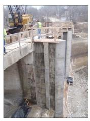
Phase 1 Status: First photo— Lunda has finished placing rebar and forming new south Dam Pier Nose and pored back using 20 CY of 4000 PSI concrete. Sub-contractor Chosen Vallev was on site to sample and test concrete. Finished removing bad concrete on Operating Deck at Dam Piers and Abutments. After Concrete Condition Survey has continued on Wing Wall at south side of Stilling Basin, saw cut-
