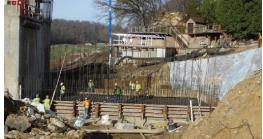
the new North Dam. Shows how far concrete is being pumped for North Dam construction. April 14, 2015, was a historic event in the life of Lake Delhi. The new North dam portion of Phase 1 had its first concrete pour. Approximately 162 cubic yards of concrete were placed in this one
