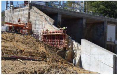
This picture above shows a close up view of forming and and rebar placement for north wall of new spillway.
