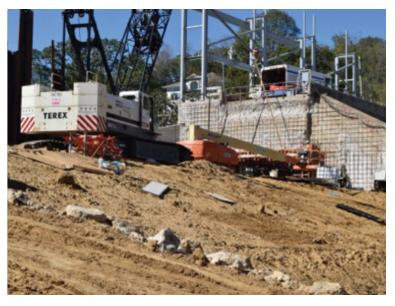
In this picture above, GCI's 100 ton crane is sitting on top of the completed earthen dike. The new spillway and earthen dike will be in excess of 40 feet high when complete. This picture gives some of this perspective of the size of this new dike and spillway. Currently GCI
