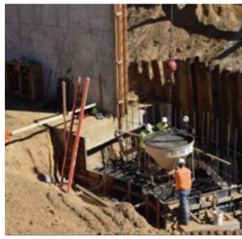
Picture below shows the far concrete wall on the north side of the new Phase 2 spillway work. The original buttress wall was extended and the former south face of the concrete powerhouse
