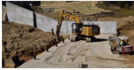
of stilling basin between the two walls. The back hoe on the left is jack hammering into bedrock to form a structural trench for the toe of the sloped concrete slabs that will cover the entirety of the earthen embankment. The smaller back hoe on the right is preparing the end of the spillway for rip rap that will extend the erosion control for the water exiting the new spillway.
